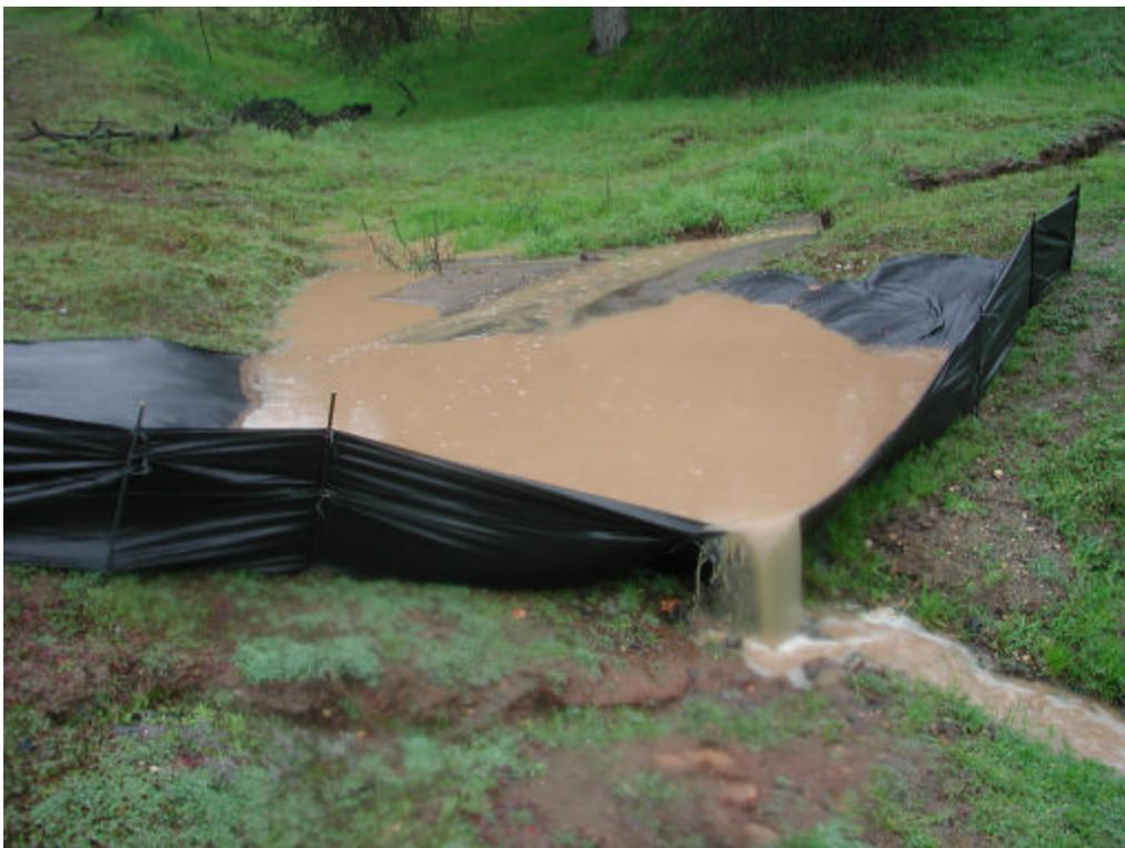
A sediment trap has been used to measure soil erosion and sediment production in the watershed.
