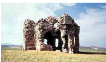
Kumbet kilise, all facing stones removed
