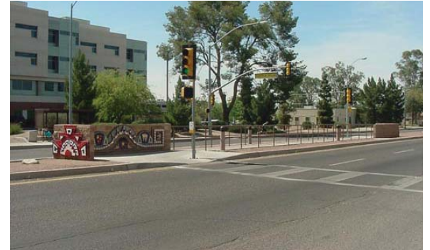
Figure 5-22: Pedestrian Light Controlled Crossing
