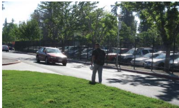
Figure 5-25: Lack of sidewalk along Scott Avenue
