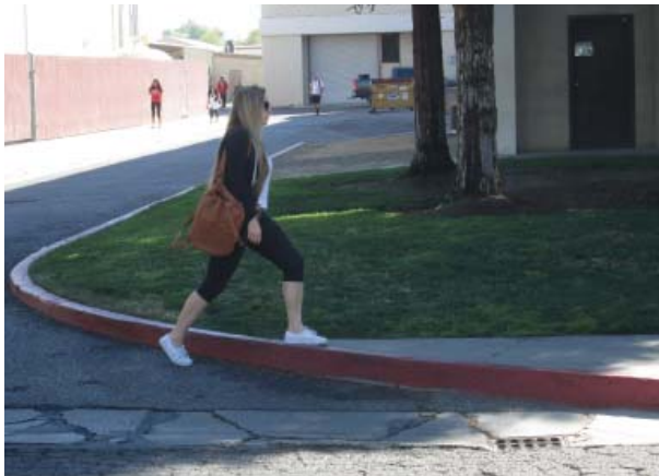
Figure 4-4: Students must step up onto sidewalks at several campus locations, limiting ADA access
