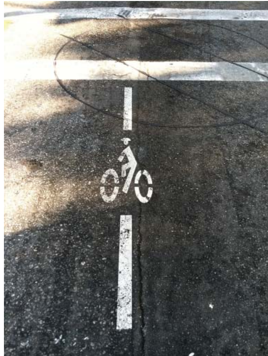
Figure 5-12: Bike detection marker at traffic signal
