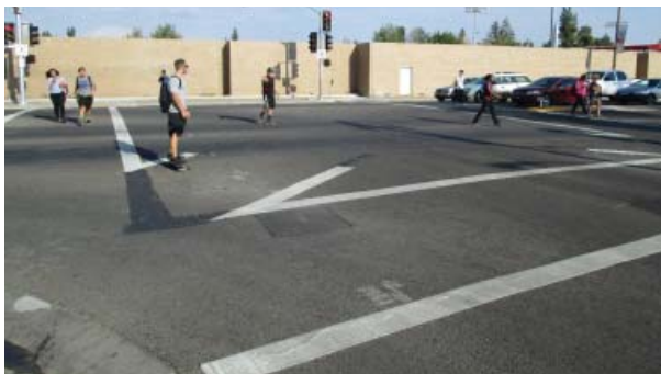
Figure 5-18: Pedestrian scramble at the Cedar Avenue/Bulldog Lane intersection
